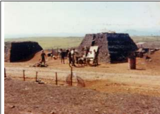
Improving bunker at entrance gate
