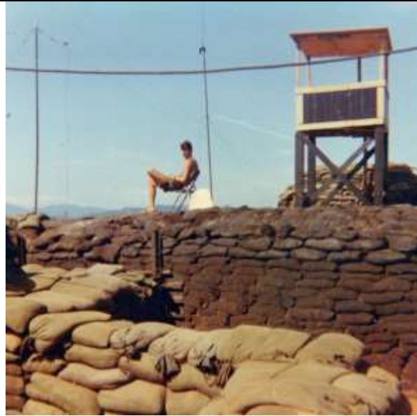
Sandbag wall provides extra protection
