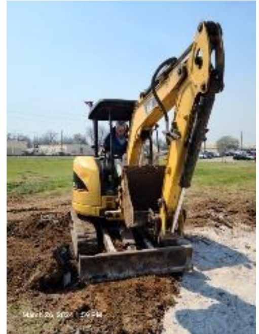
Jackie Carver laying down the crushed rock sub-layer.
