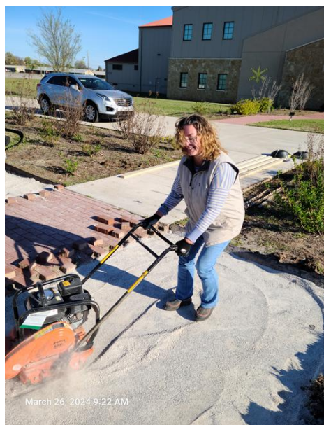
Melita Simily takes control of the soil compactor on the stone bed.
