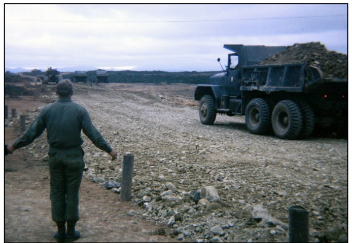
Building Dong Ha Combat Base.
