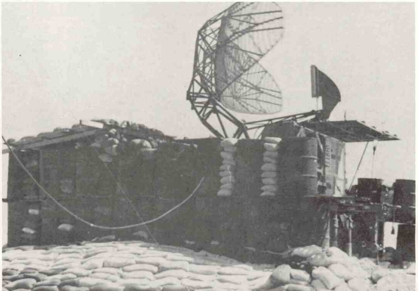
HAWK positions resembled sandbagged fortresses. During the monsoon, trenches dug through the fortifications turned into moats.
