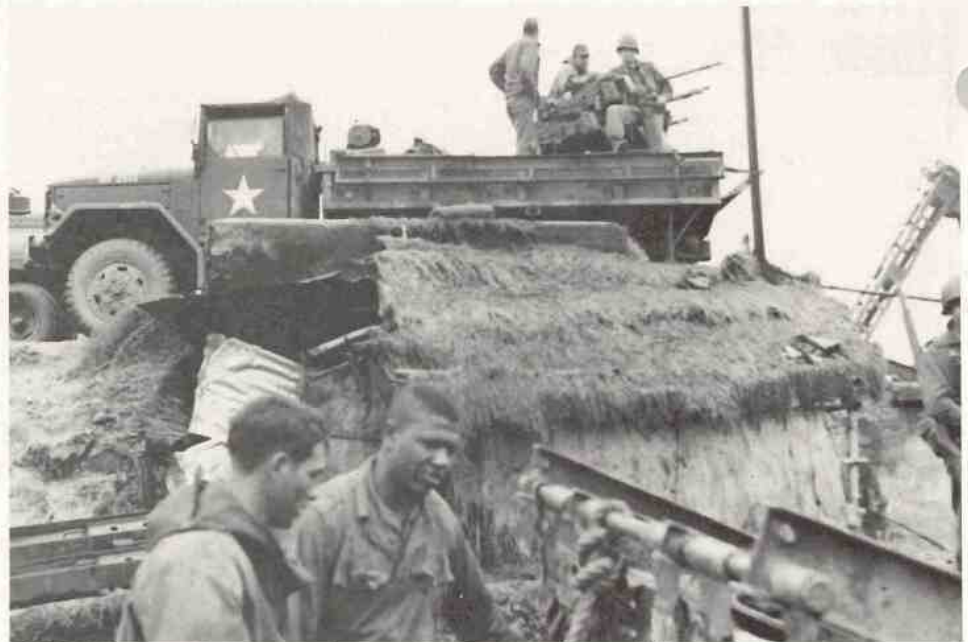
QUAD 50s were often mounted on trucks to increase their mobility.
