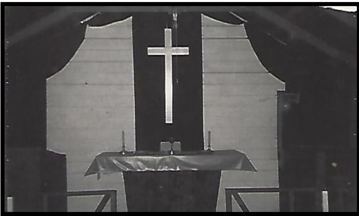
Newly constructed Chapel at Qui Nhon
