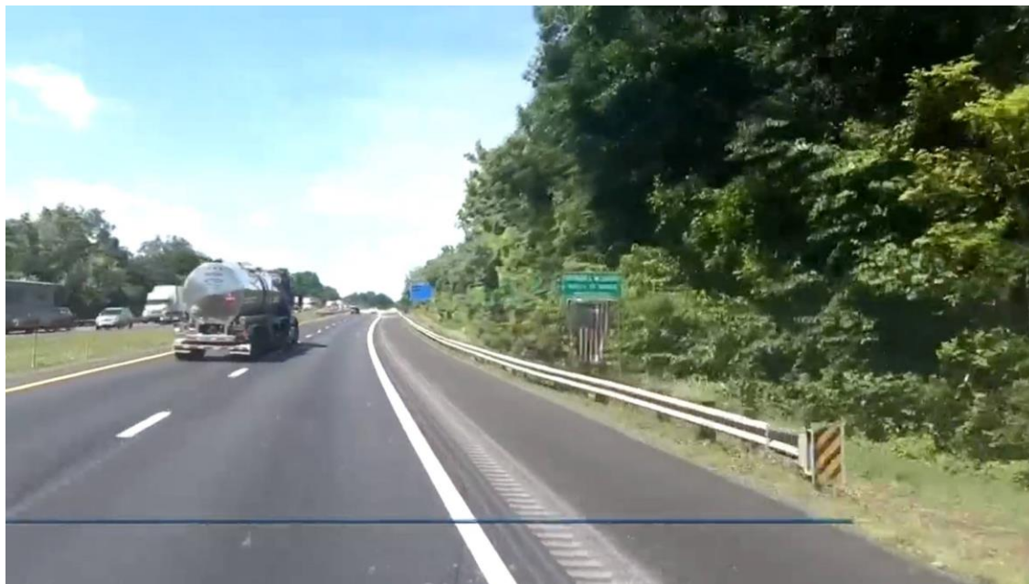
Figure 2 Stout MOH bridge on Interstate 75 in Loudon County, TN -sign
